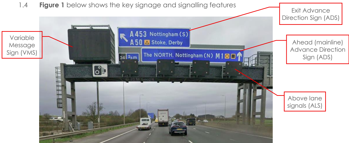
Figure 1: J24 Primary ALS/ADS/VMS gantry with features labelled (image courtesy of Google).
